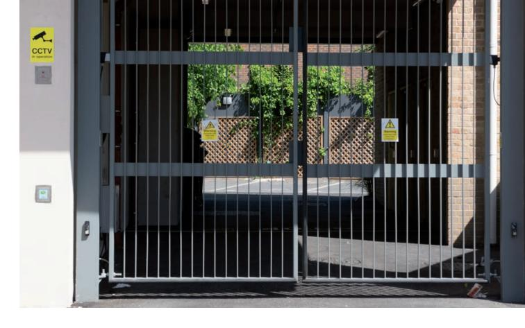
Right leaf of vehicle gate opens when proximity reader is used by cyclists, both leafs open when radio transmitter is used by motorists. All controlled by the IPGUARD® smart system and remotely programmable!
